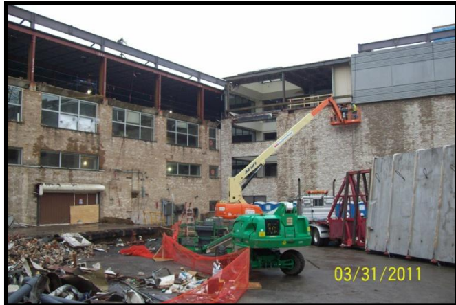
Demolition of Existing Parapet for Perimeter of Main Building
