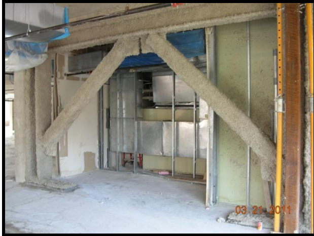
Installed Seismic Bracing
