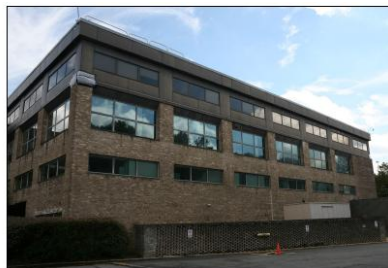
Southwest Building (red arrow)
