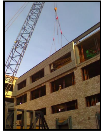
Precast Panel Installation
