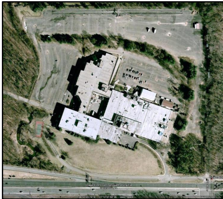
Existing 7700 Arlington Blvd. Site
